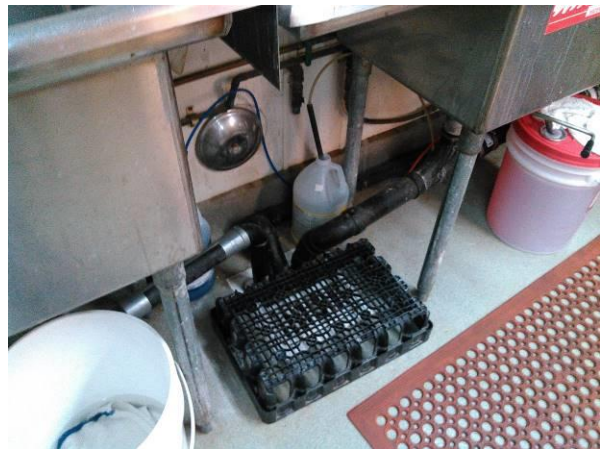
Photo 16 View of a typical kitchen floor drain.
