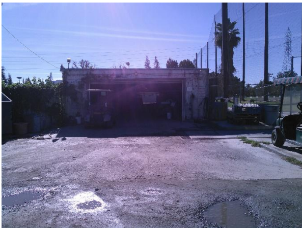
Photo 15 View of the cart wash area and sump looking south.
