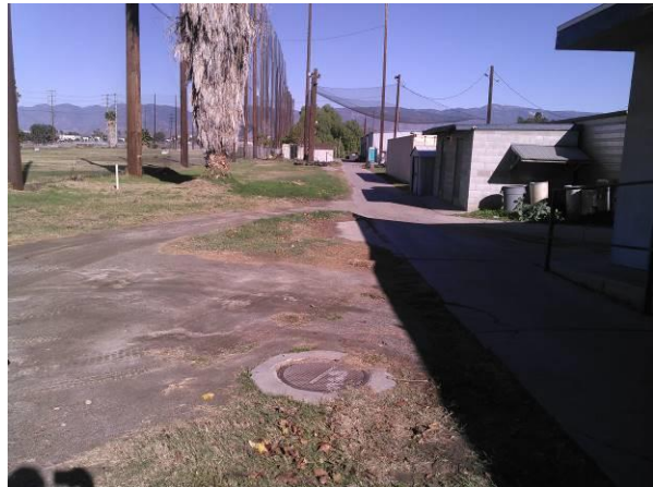
Photo 8 View of the western septic tank and leach field.
