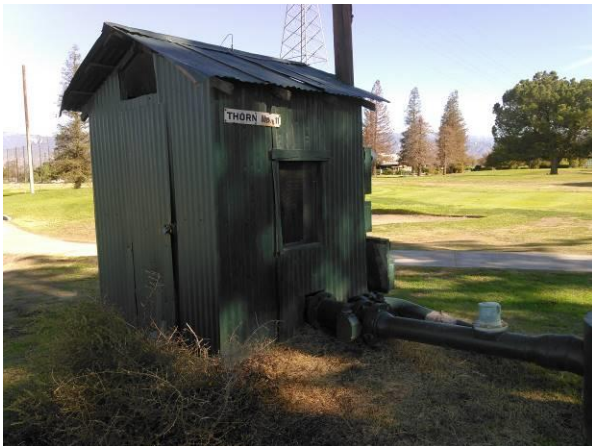
Photo 11 View of a groundwater production well.
